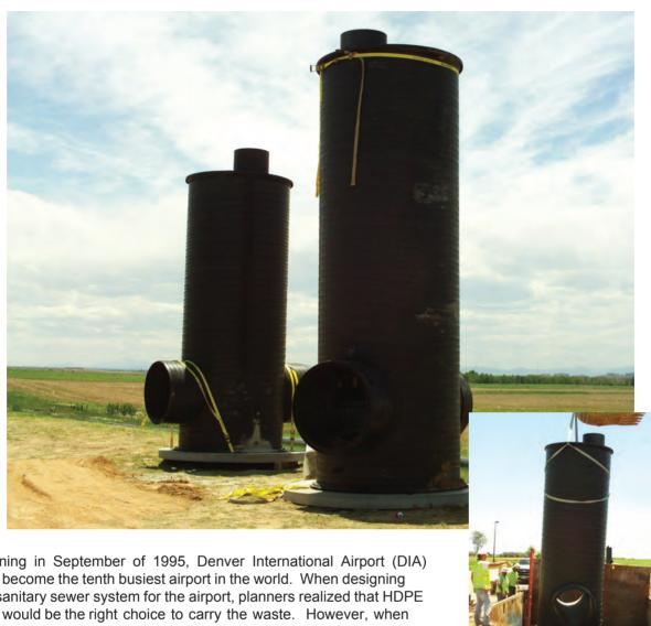
Opening in September of 1995, Denver International Airport (DIA) has become the tenth busiest airport in the world. When designing the sanitary sewer system for the airport, planners realized that HDPE pipe would be the right choice to carry the waste. However, when designing the manholes, they believed plastic lined reinforced concrete manholes would also be the right choice. This turned out to be wrong.
